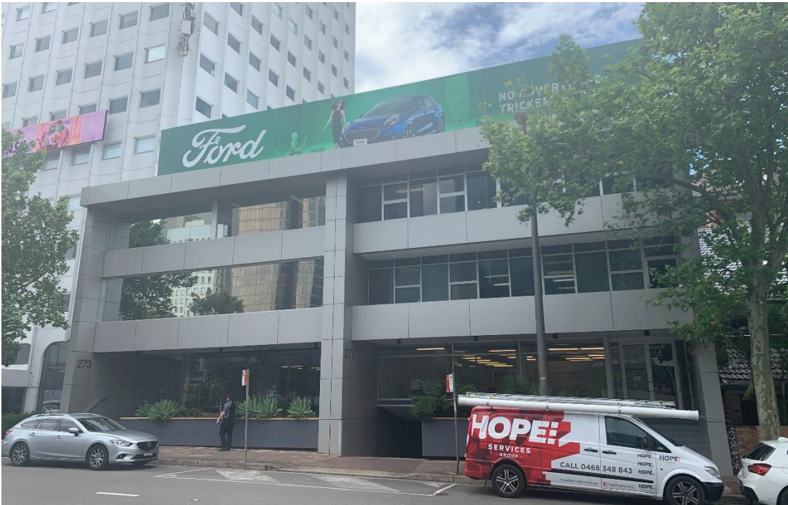
Figure 10 – 271-273 Alfred Street, principal frontage.
