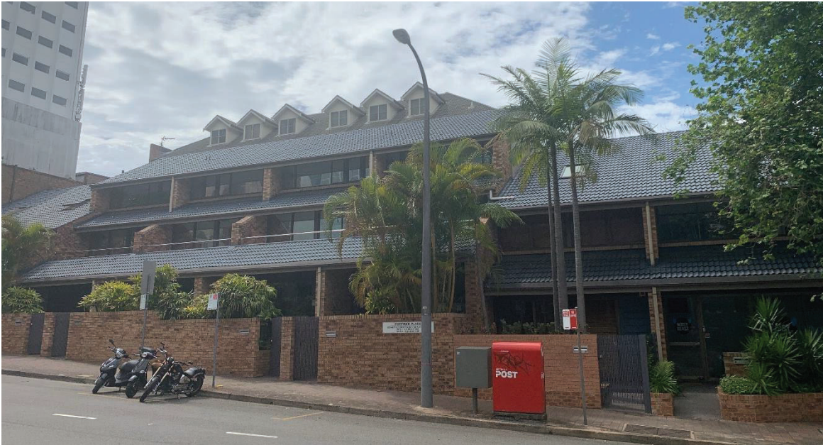
Figure 8 – 263-269 Alfred Street, principal frontage.
