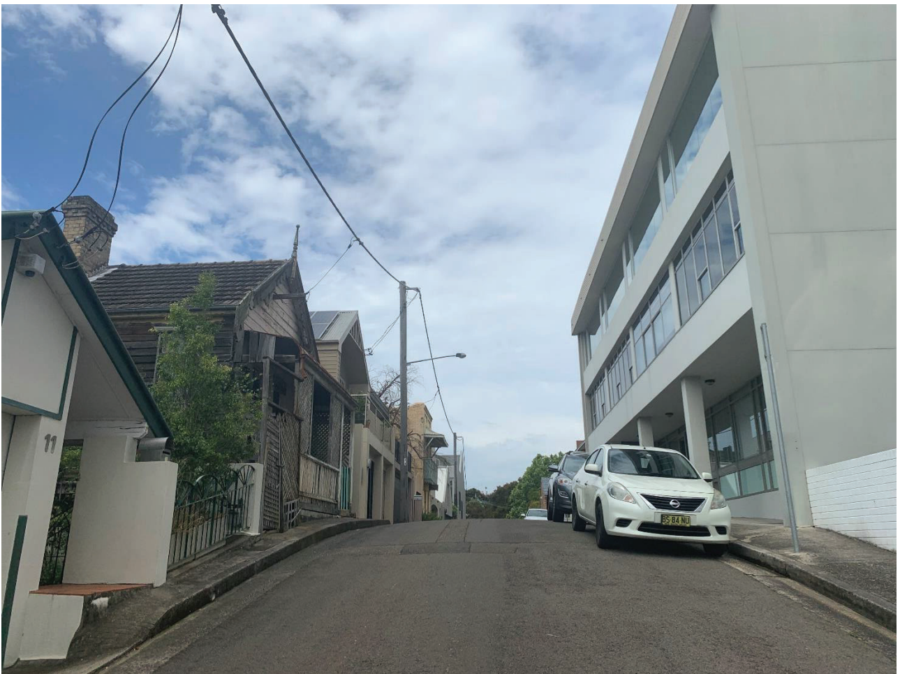
Figure 7 – View facing south along Little Alfred Street. Subject site is at the right of image; low-scale residential development, within the Whaling Road HCA, is at the left.
