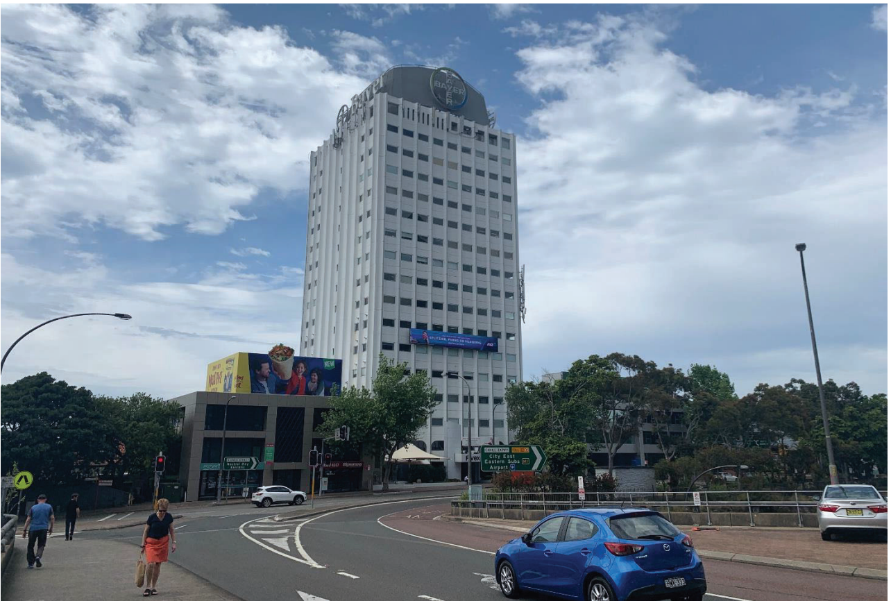
Figure 5 – View facing north along Mount Street towards subject site.
