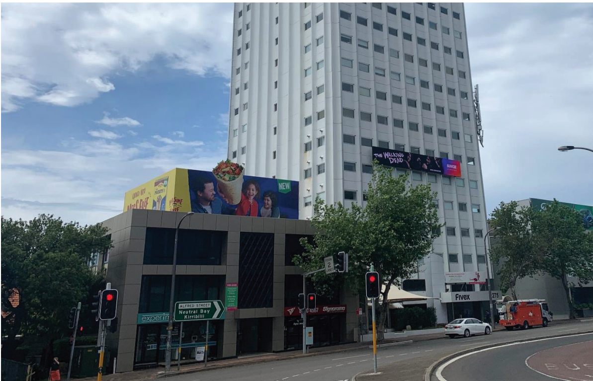
Figure 13 – 283 Alfred Street, principal frontage.
