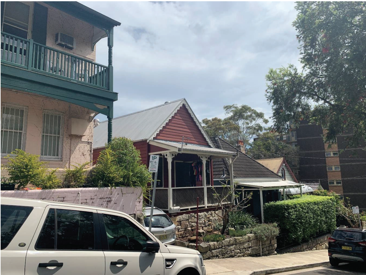
Figure 18 – View facing north along Doris Street, with listed item “Dorking” (12 Doris Street) at right of image.
