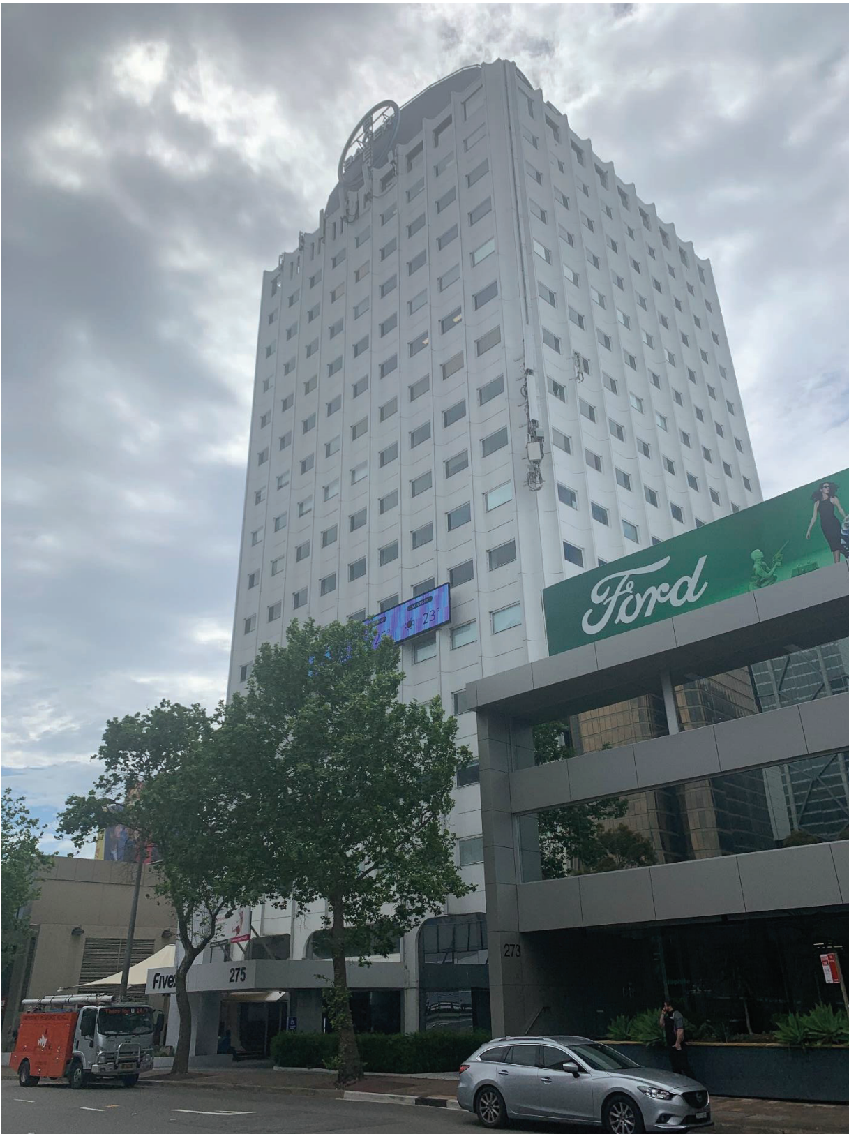
Figure 12 – The 'Bayer Building', principal frontage at Alfred Street.
