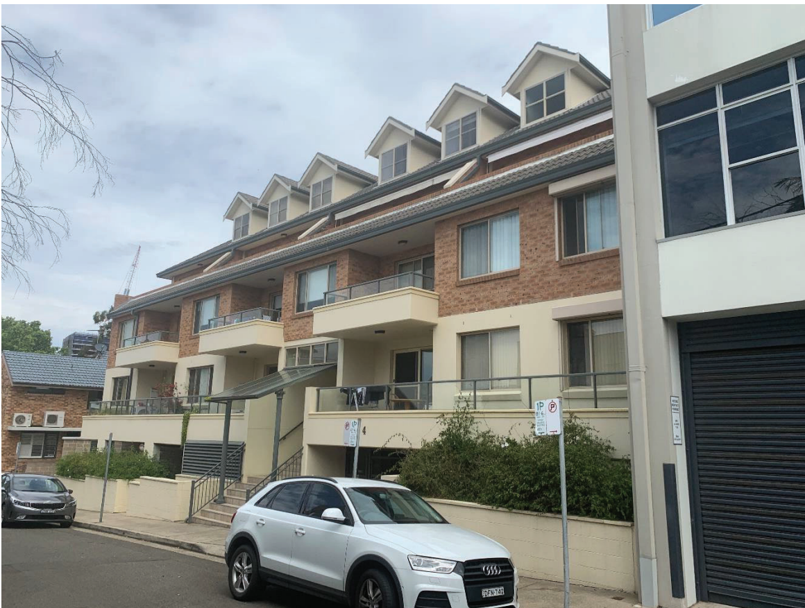
Figure 9 – 4 Little Alfred Street, principal frontage.
